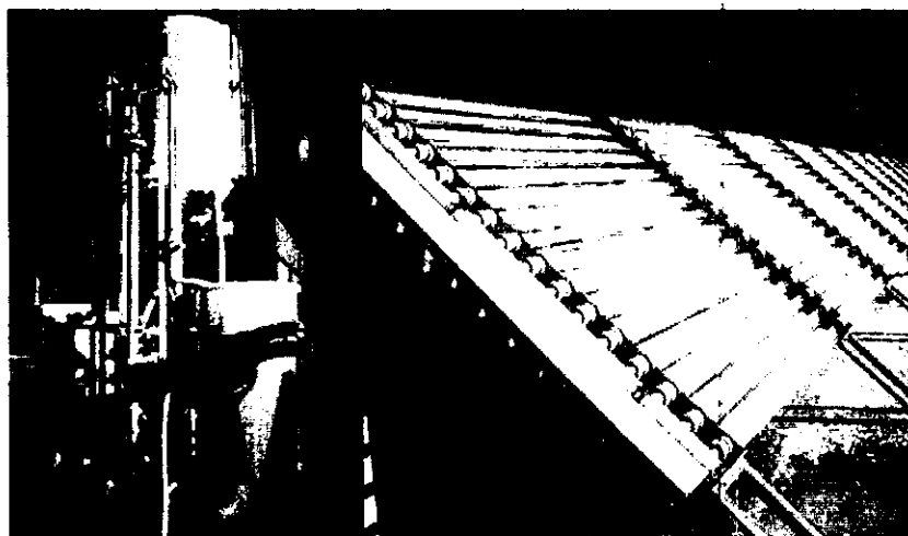
Fig. 15. Photographs of solar detoxification demonstration plant constructed in "SOLARDETOX" project at HIDROÇEN (Madrid, Spain). Left: TiO 2 separation system. Right: compound parabolic collector.
