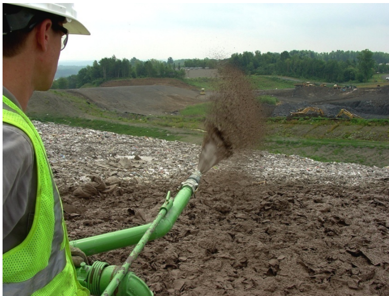
Figure 6 – Spray applied coating used for landfill daily cover (Courtesy of Landfill Services Corp)
