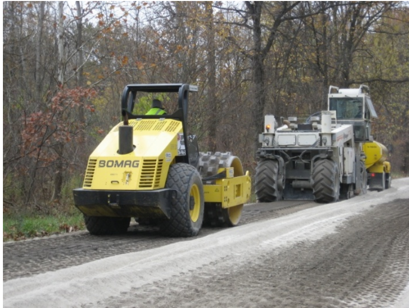
Figure 4 – Constructing a pavement base using CKD (Courtesy of Lafarge North America)
