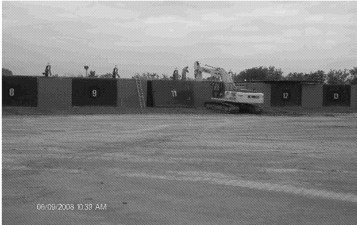
Front view of treatment cells 8 to 13. Cell eleven is being emptied: the roof and front wall have been removed.
