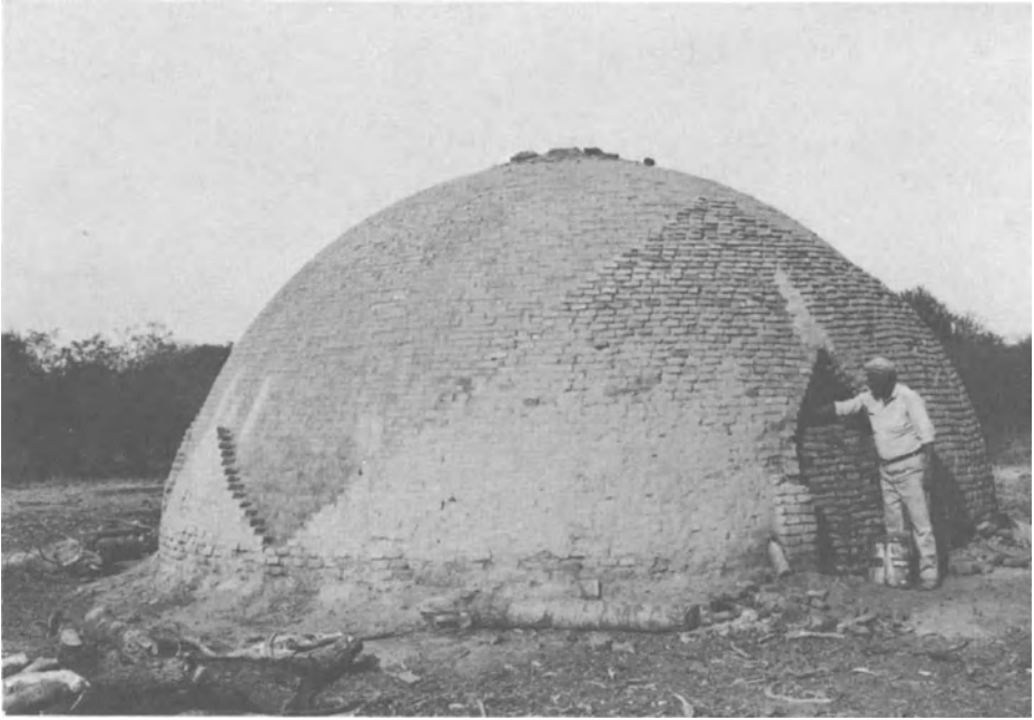
PHOTO 7 The Argentine half-orange kiln. The operator is closing the gate after charging the kiln. (Photo W. Emrich)
